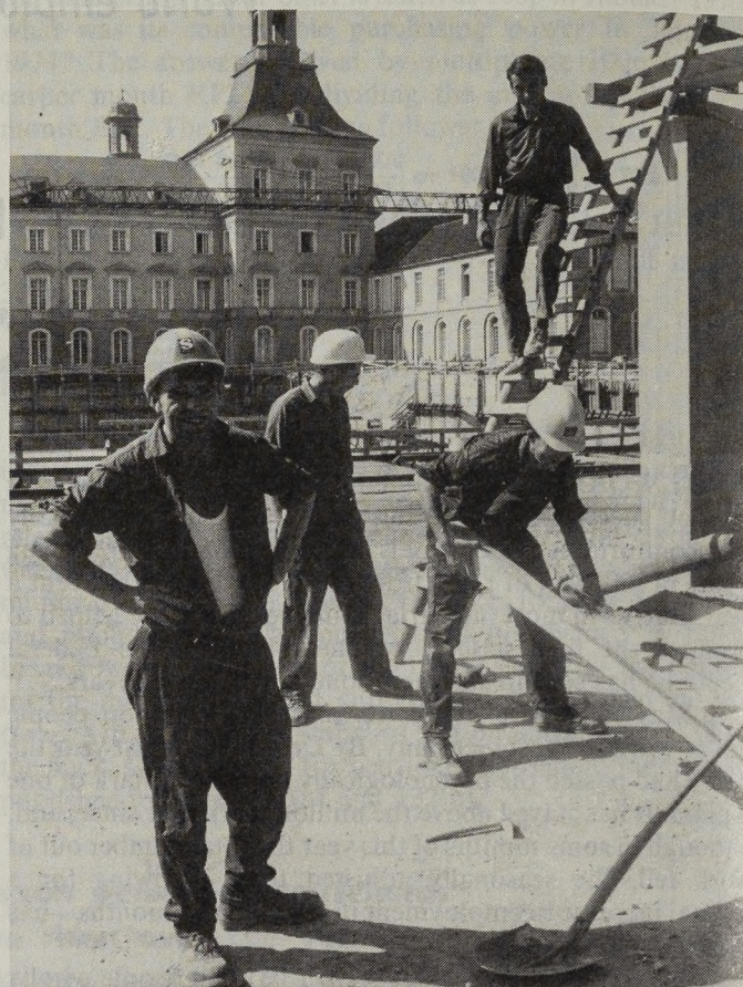
Yugoslavian "guest" workers on a building site in Bonn.
