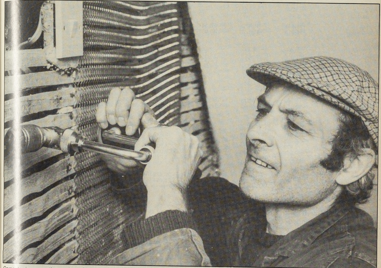
Carpenter in renovation project, Cornwall.
