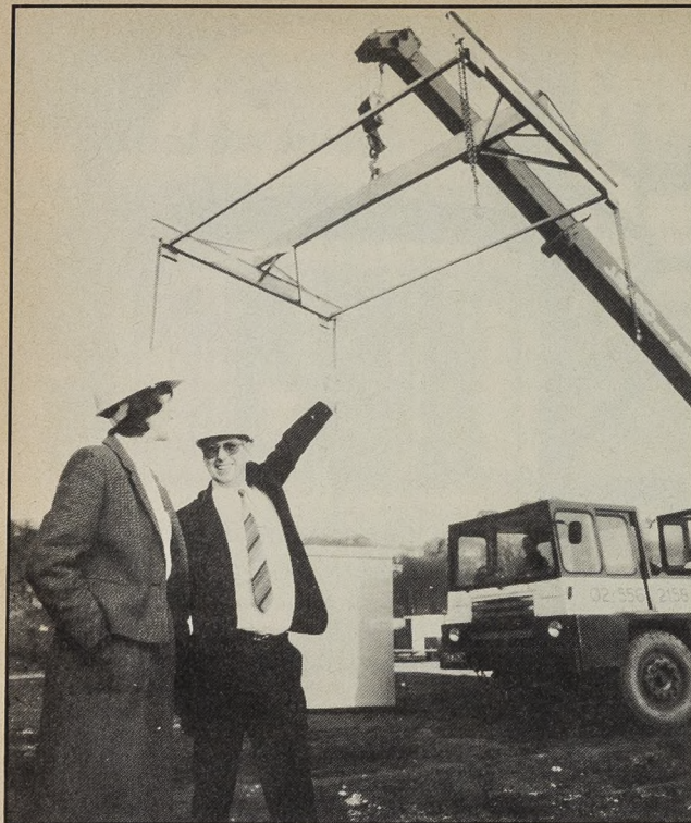
BTH Industries Ltd, Wakefield, have successfully completed their option BGT 3 project and intend continuing to employ their consultant.
