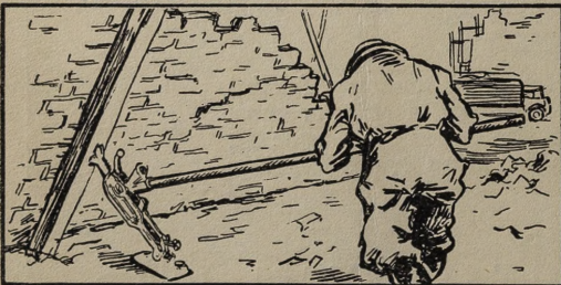
PUSHING OVER OR PROPPING UNSAFE WALLS
