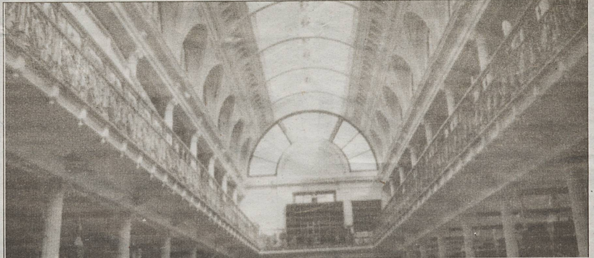
The library's final days at the Southampton Buildings are approaching
