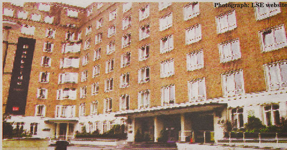
It emerged that the hot water shortage at Bankside House was caused by a faulty transistor
