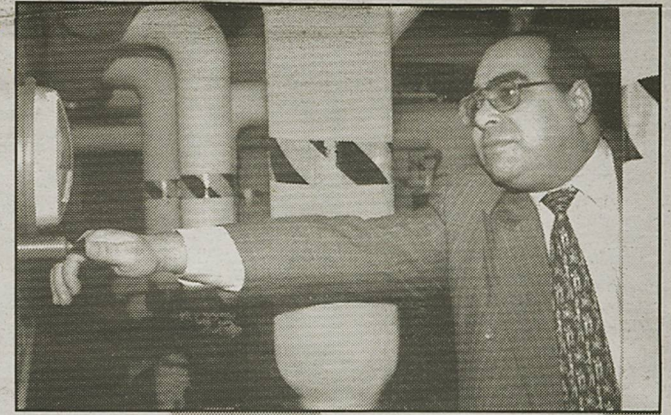
In the secret labyrinth of the theatre's basement, all lights are switched on and the oil supply and power backups are checked.
