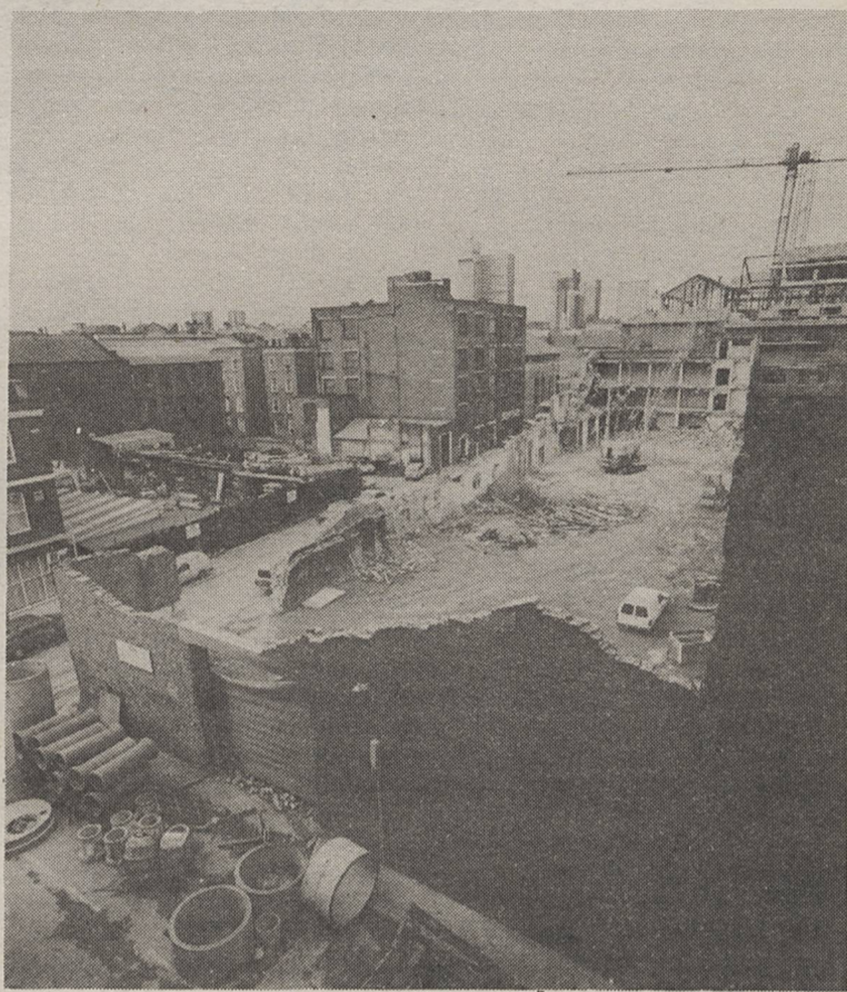
The building site at Butlers' Wharf
