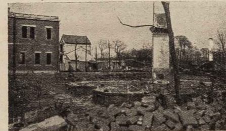
Two fire-places, much ash, scattered typewriter keys, a heap of rubble, were all that were left of the Y.W.C.A. National Office.
