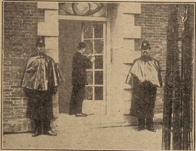
REPAIRING MR. MCKENNA'S HOUSE.
