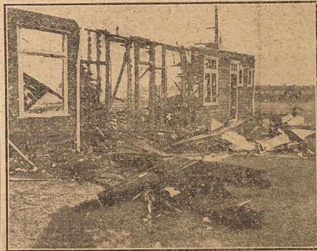
RUINS OF THE CATFORD PAVILION.
