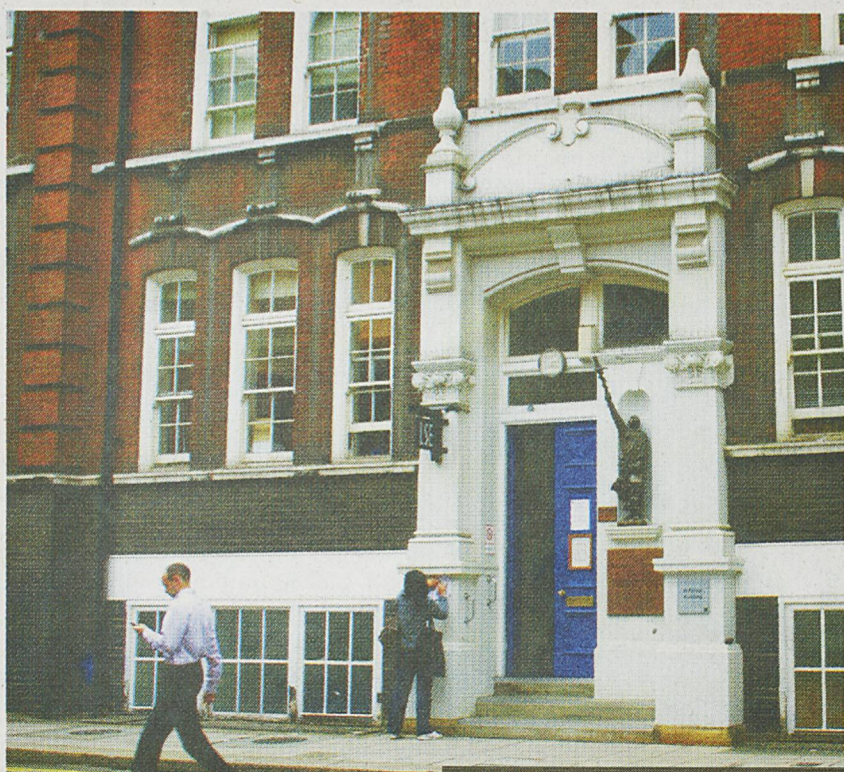
St. Philips building, due to be demolished Photo: Beaver archives
