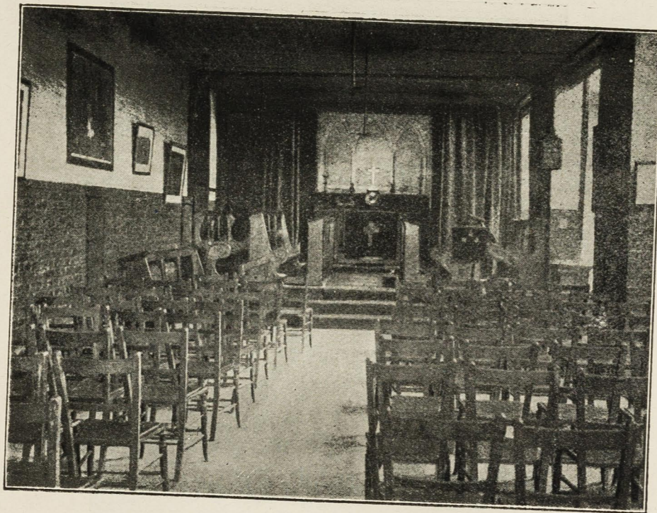
Trinity Mission Building, Albany Road.
