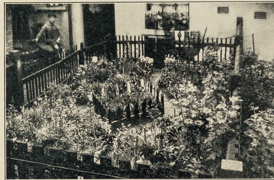
Talfourd Street Property after Reconditioning by Copec Society.
