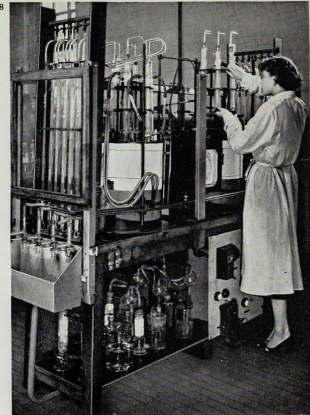
An oxidation test being carried out on insulating oils
